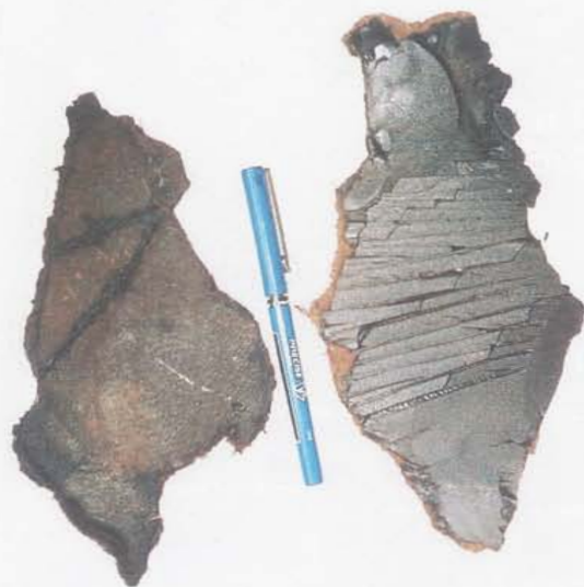
Figure 1: Samples of coating with possible asbestos presence.
